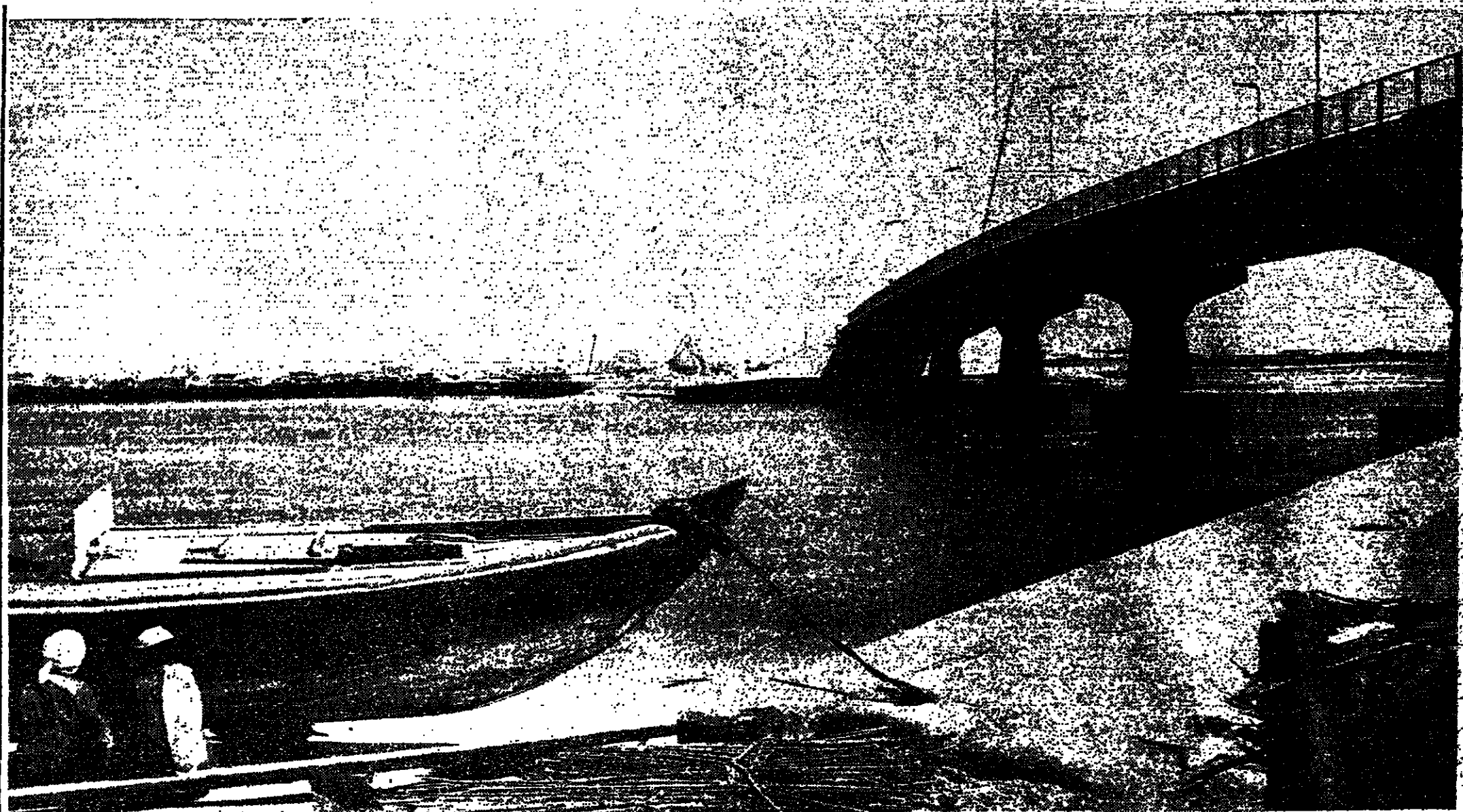
The fine new bridge across the Creek at Dubai. A tunnel is also being dug near the entrance to the Creek to filter off some of the rapidly growing commercial and domestic traffic.
